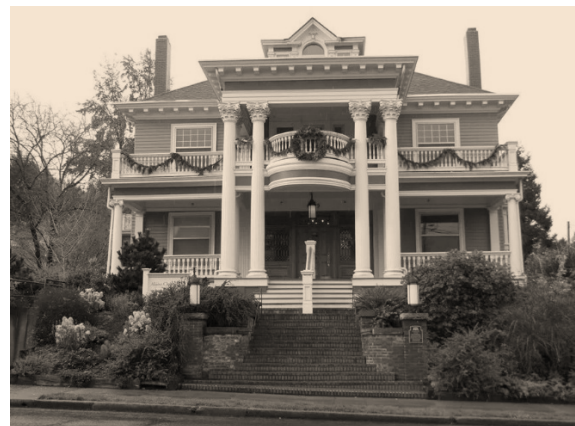
Portland Alano Club est. 1947, 909 NW 24th Ave, Portland
